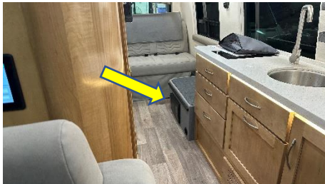
Locate Fuse Panel
