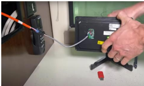
Remove Touch Screen from wall
